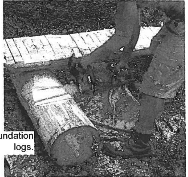
Cut selected timber at McCann Farm and prepare log with adze.
